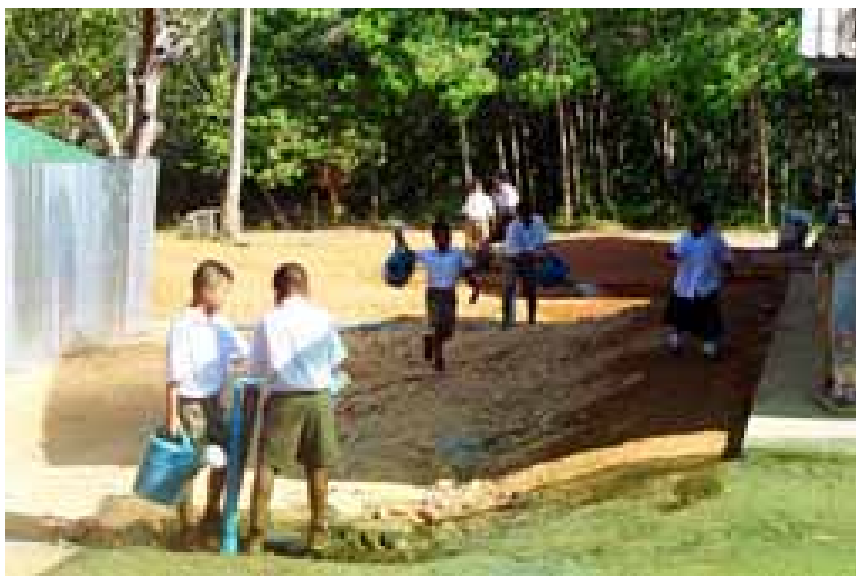
Watering the ground to keep the dust from the construction out of the temporary school.
